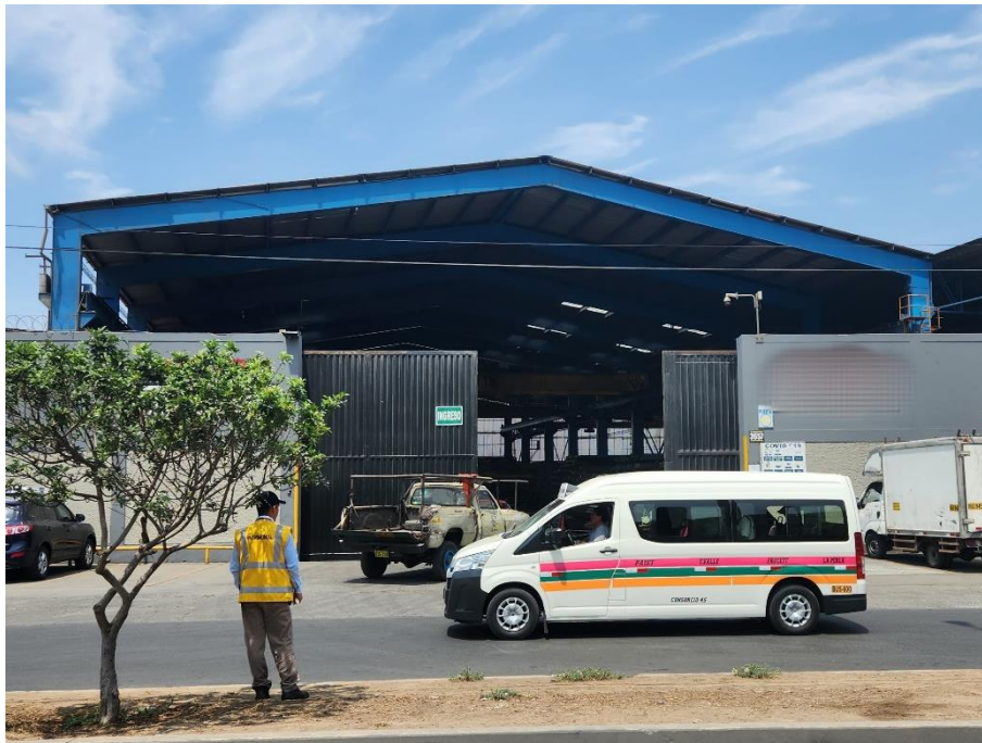
Figura 36. Estructura industrial (IC).
